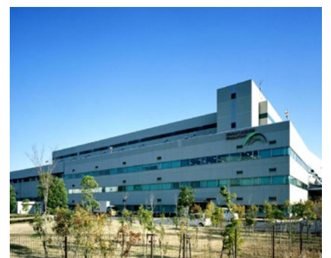
Narita, Chiba, Japan, storage/logistics building
