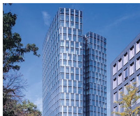
WestendDuo, Frankfurt/Main, Germany, office building
