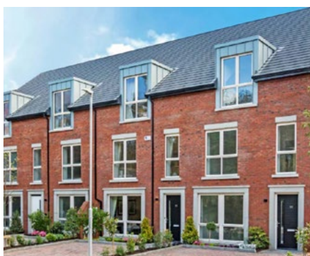
Cedarview, Santry, Ireland, residential building
