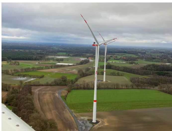
Wind farm, Ostbevern, Germany
